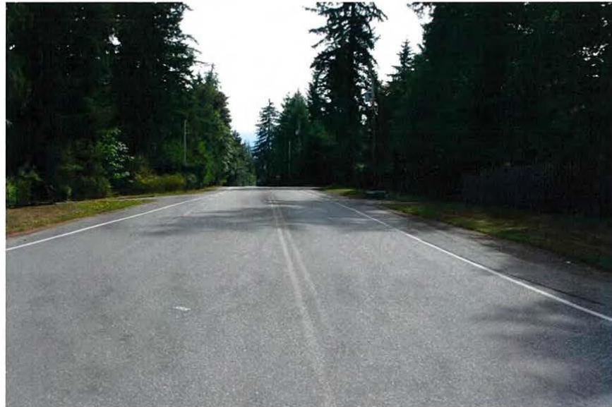
Exhibit 2 – Faded road markings on Forbidden Plateau Road approach to Piercy Road
